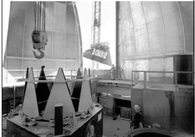
Construction of the Kitt Peak National Observatory's 2.1-meter telescope, dating from 1960.
